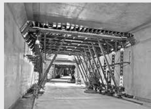
Tunnel Formwork
