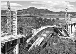
Bridge Formwork
