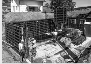
Wall Formwork
