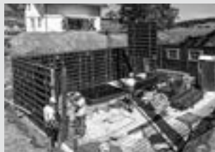
Wall formwork
