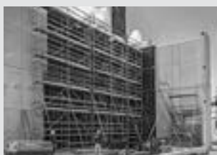
Working scaffolds construction
