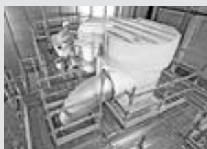
Working scaffolds industry
