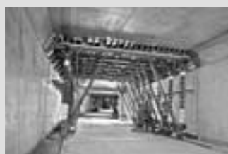
Tunnel Formwork
