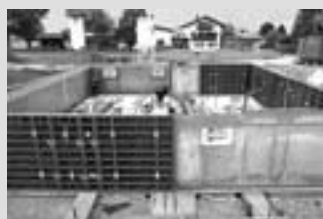
Wall Formwork
