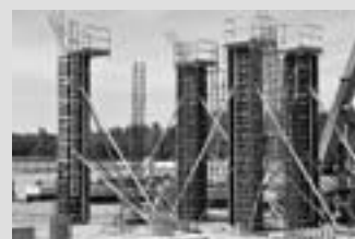
Column Formwork
