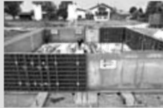
Wall Formwork
