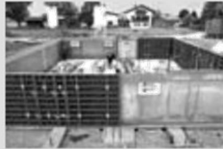
Wall Formwork
