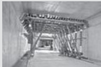
Tunnel Formwork
