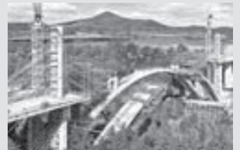
Bridge Formwork
