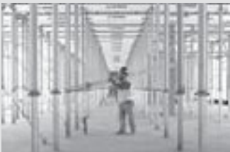
Slab Formwork
