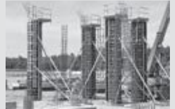
Column Formwork
